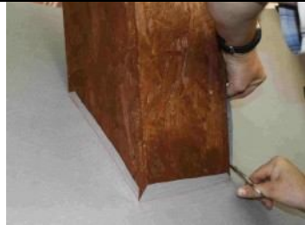
10.4 trim the triangular edges around the chimney
